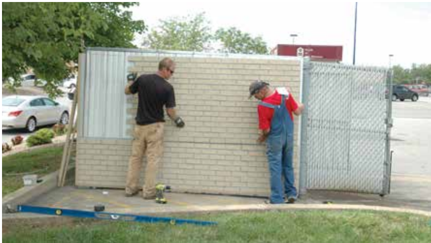
Taking down the chain-link fence enclosure (above) and putting up brick (below). First the fence is removed; then a frame is built and bracket installed on the four posts. Next comes a modular frame, followed by brick panels. The process takes less than a day.
